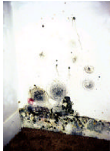
An example of mold in an extremely advanced stage.
